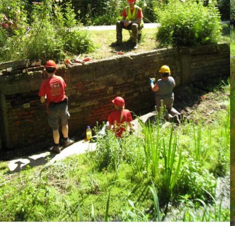
A visiting group undertook piling and brickwork repairs on the Deepcut flight (2012)
