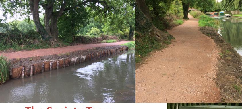
The Society Team repaired the bank and paved along 100m of towpath at Colt Hill, and also installed a new water point at the Canal Centre (2017)
