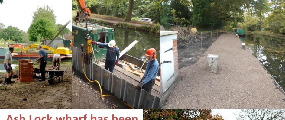
Ash Lock wharf has been enhanced with the installation of a new water point and piling and paving of the bank (2019)
