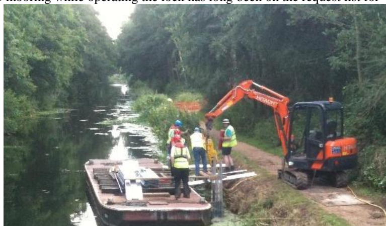
Members of the WRG team constructing the mooring below Lock 1.
