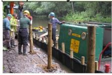
The regular Society work party has continued work at Frimley Lodge Park and have now installed soft bank protection along a 200m section of towpath as far as the model railway buildings (*left*). Construction of a 40m landing stage near Guildford Road bridge has
