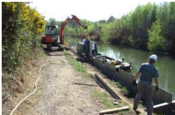
*Installing piling for a new landing stage at Runway's End, Rushmoor*
