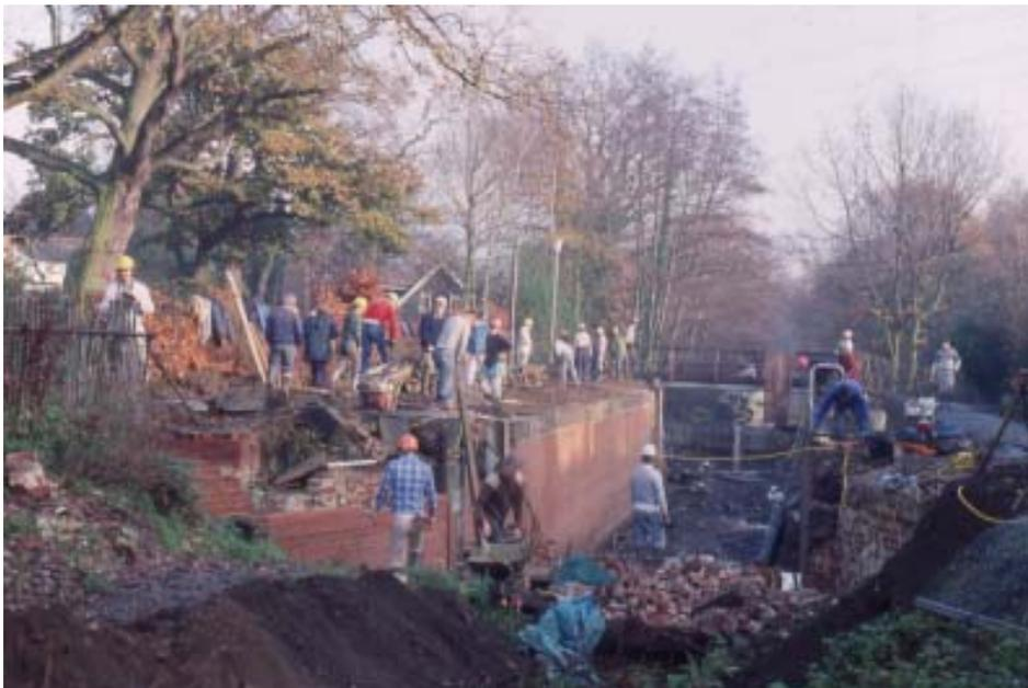
Lock 3 was the last lock to be restored; installing a bypass channel was particularly difficult. The scene above was probably taken in 1989. The picture below shows it fully navigable again.
