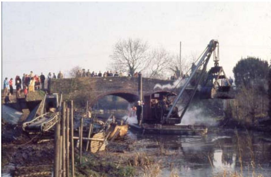
While most of the canal was dry dredged using excavators, the stretch from North Warnborough to Pondtail in Fleet was dredged by a 50 year-old steam powered dredger “Perseverance”. The job started at Colt Hill in 1976(*above*). A miniature railway was used to carry away the silt (*below*).
