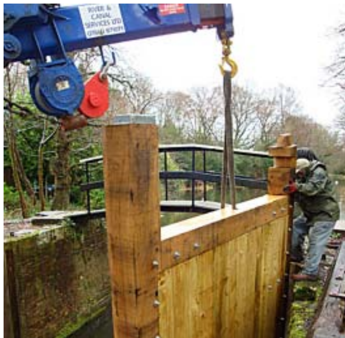
Above: Rob Locatelli's men installing new gates on Lock 5.
