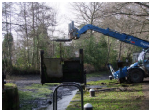
Above: The gates of Lock 13 being removed prior to being measured to ensure that the new ones fit properly. Inadequate measurements led to trouble fitting the new gates on Lock 12, so no chances are being taken. The order for the new gates has been placed with high priority.
