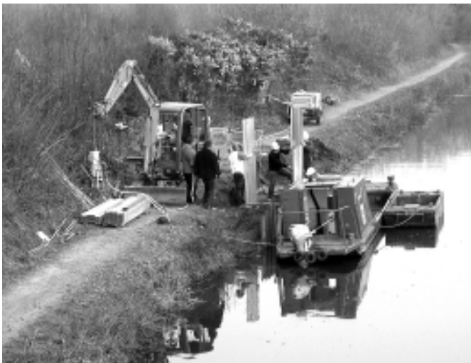
Above & below: Pile driving at Runway's End.
