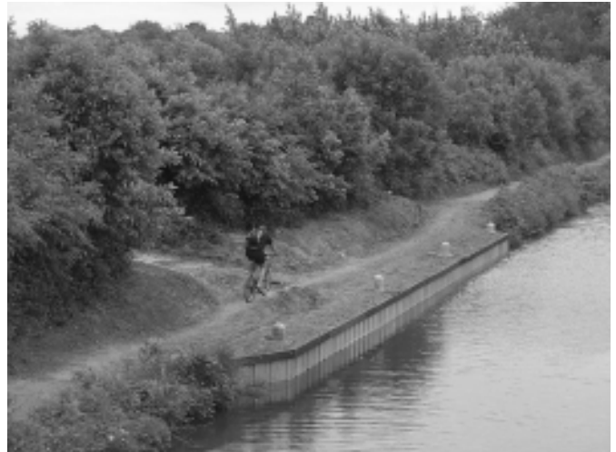
Above: The mooring almost complete with only a wooden capping strip and a layer of road stone left to do.
