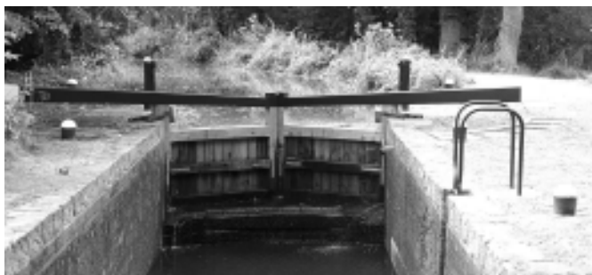
Above: New gates recently fitted to Lock 8
