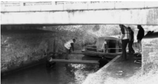
Above and top right: The first set of stop planks going in at Chequers Bridge on 1st March
