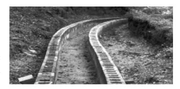
Construction of a new open channel bypass at lock 27 was completed in October (*above*) replacing an old underground concrete pipe that was prone to fracture and collapse.
