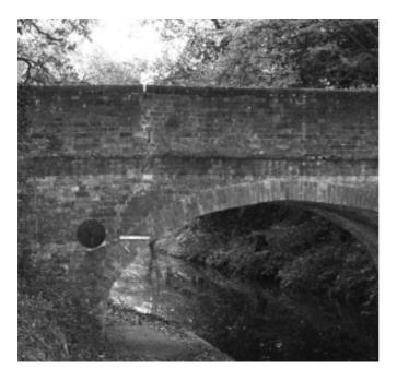
The crack can be clearly seen on the Odiham side of the bridge (*above*) and is just as bad on the other side, although partly masked by ivy. The abutment on the towpath side seems to have dropped back, and there must be great stress on the bottom of the arch.
