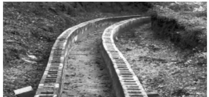
Construction of a new open channel bypass at lock 27 was completed in October (*above*) replacing an old underground concrete pipe that was prone to fracture and collapse.
