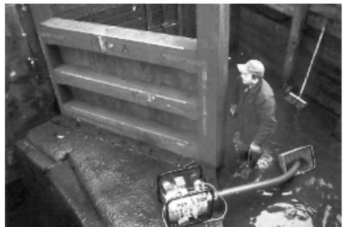
A new upper lock gate (*above*) made by our rangers is fitted at lock 11 and is a perfect fit! In future gates will be made to order by external suppliers but fitted in-house as part of a scale of economy and in order to meet the gate replacement program.
