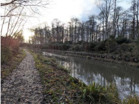
Ground anchors opposite the towpath
