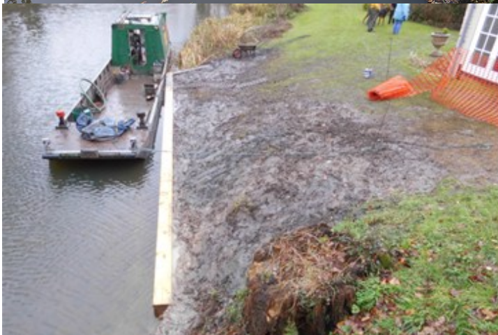
Bank reinforcements at Crookham.
