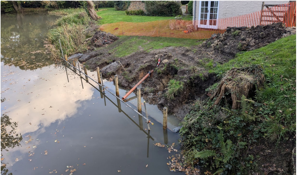
Bank reinforcements at Crookham.
