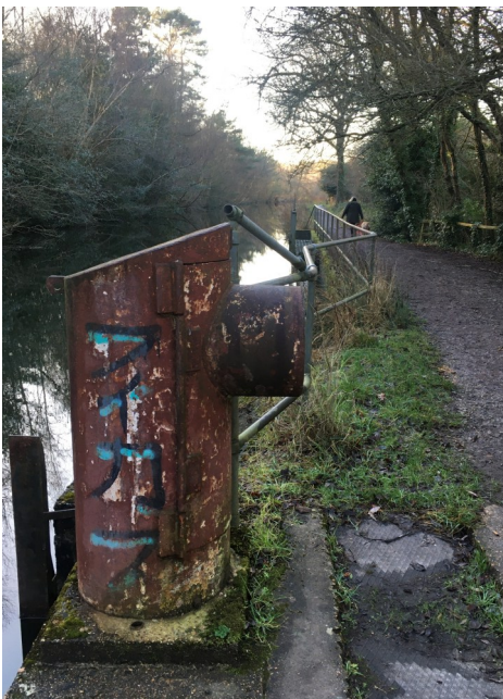
The only remaining evidence of the pumping station to Pyestock from the canal.
