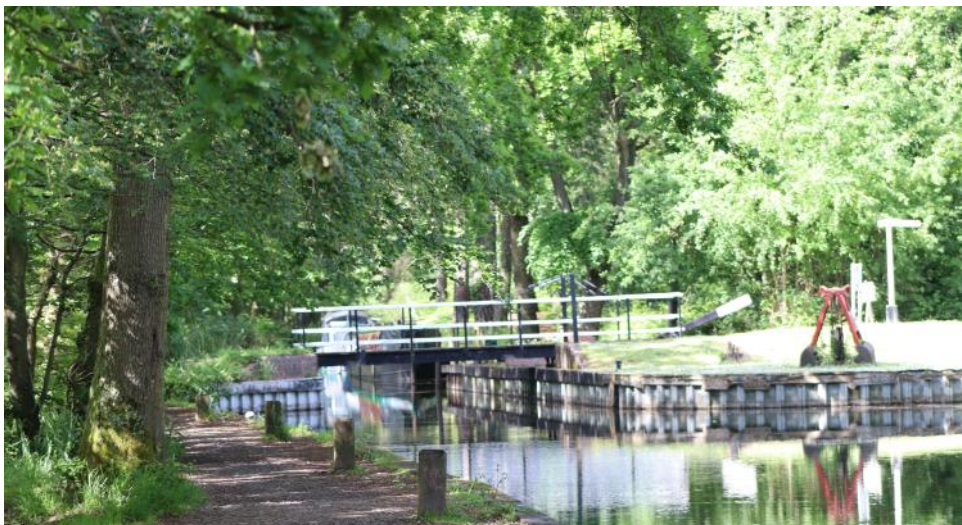
Swing bridge next to Basingstoke Canal Centre, Mytchett
