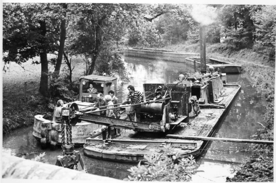
Dredger and team clearing the mud: 1980
