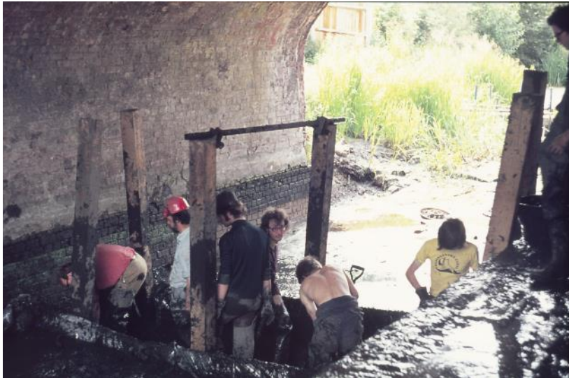
Digging out the canal after it had fallen into disrepair
