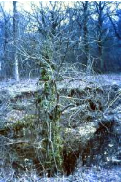
Hole in ground above Greywell tunnel roof fall. 1966
