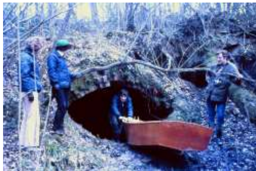
Greywell Tunnel exploration, Western Portal, 1966
