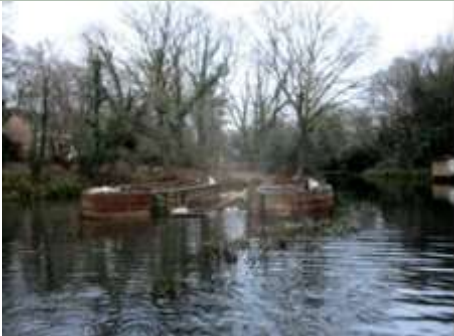
End of first wet weekend barge lifting
