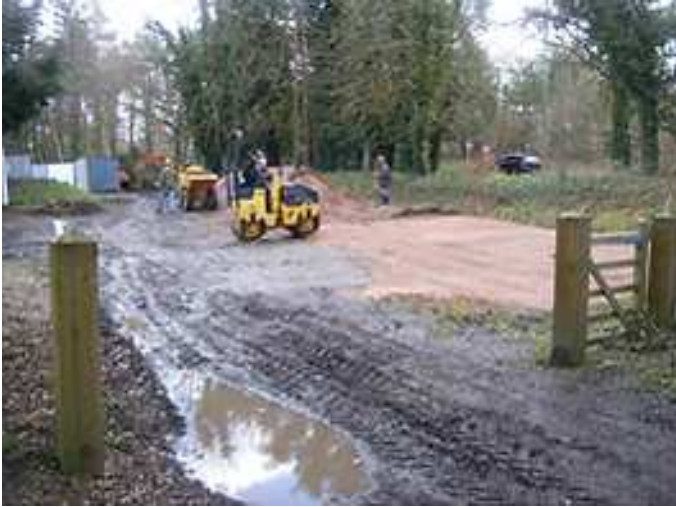
Laying roadstone on the second car park
