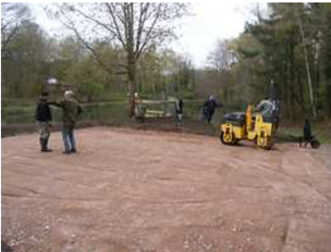
Above: The new Canoe club base & the now small viewing area
