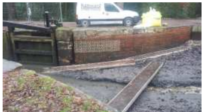
Below: Upper wing wall patching
