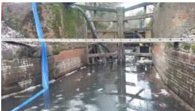
Above: Gates ready for re-planking
