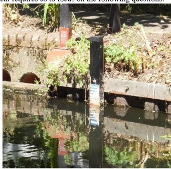
that discharge water from the canal during wet weather thereby preventing flooding.
