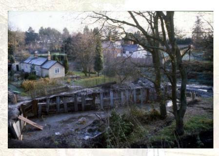
This seemed excellent idea, so work began. The dock was completed by the autumn and the Society's trip boat, John Pinkerton, underwent its first outof-water hull inspection there in September 1984. The supports on which a boat sits to enable access to the bottom of the hull were originally a temporary bridge that the army
