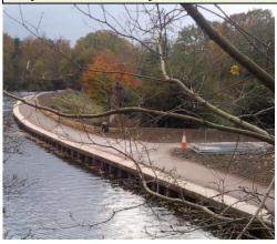
The imminent completion of the <u>repairs</u> to the <u>Mytchett</u> <u>embankment</u> (*left*) was reported in the <u>last Bulletin</u>. Some more work still has to be done, including laying a membrane over the towpath to prevent it retaining water (which might cause the
