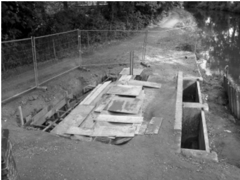
Left: The nearly completed pump chamber below Langman's Bridge.
